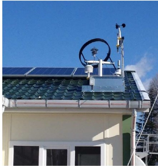
(a) Placement of measuring sensors.
